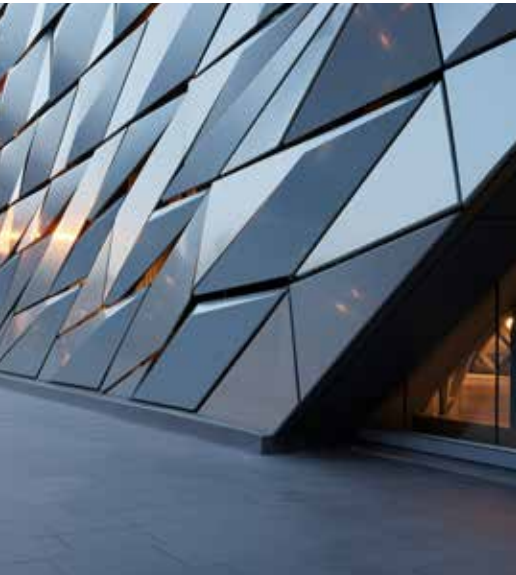
Decorative curtain wall
